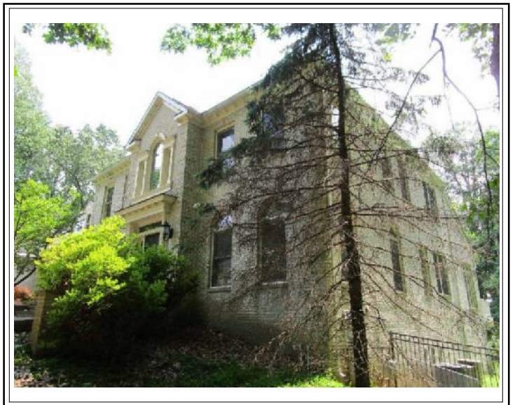
Additional Front Photo #2
