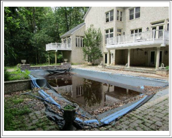
In-Ground Pool - Photo #1
