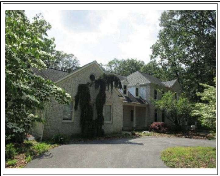
Additional Front Photo #1
